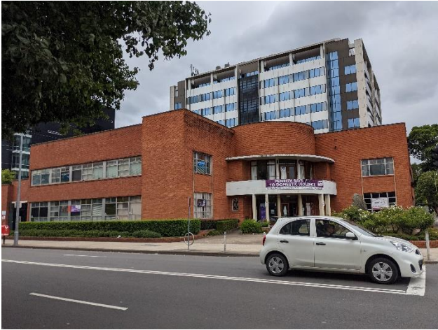
Figure 10 – Former Penrith Council Chambers
