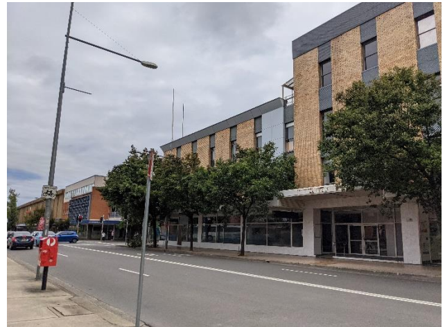
Figure 13 – Eastern façade of Borec House viewed from Station Street
